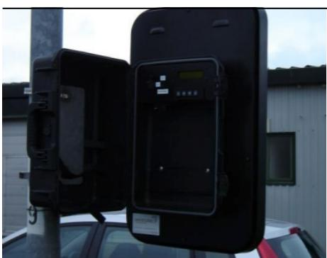
Open the sign and place the battery inside. The sign is now installed and ready for operation. Connect the solar panel to the sign using the provided plug. Secure the bracket, sign, and solar panel with padlocks.
