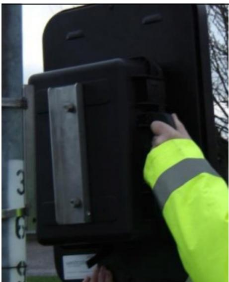
Carefully lift the sign onto the bracket. The sign has two nuts that fit into the keyholes on the bracket. Once fully inside the keyhole, slide the sign down into the smaller part of the hole. When this is completed, the sign will be securely in place.
