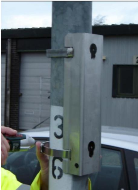
Make sure that the bracket is installed with the keyhole cut-outs as shown facing outwards; the larger part of the keyhole towards the top with the smaller towards the bottom.
